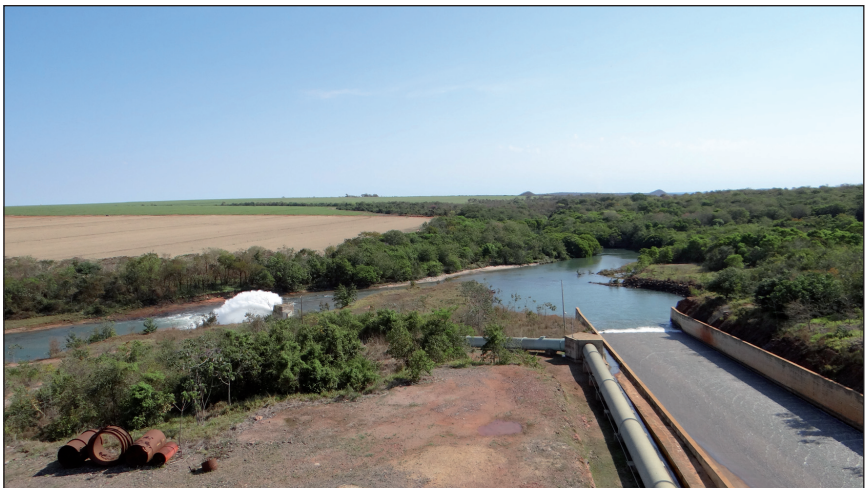
Figure 3 - Spillways of the Ponte de Pedra HPP and the natural channel of the Correntes River. In this section of \sim 12.7 km length, the flow comes exclusively from water releases of \geq 9.7 \text{ m}^3/\text{s} (August 2016)
